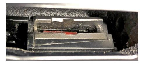
As you can see in this photo, debris have accumulated inside the magazine and around the feed lips.
